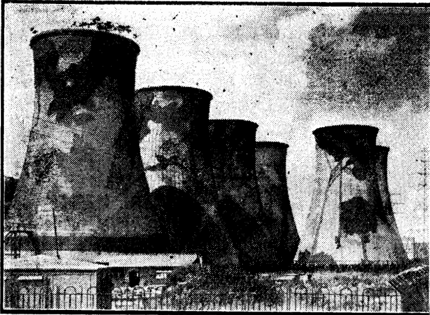
The cooling towers of the Leicester electricity power station in England were camouflaged by painting them in suitable colors and "decorating" them with tree shapes. The presence of such large structures, though camouflaged, is often betrayed to observation aircraft by the shadows cast at early morning or late evening.
